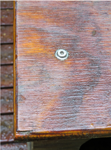
Fig. 3. Sealed Edge Fastener.
