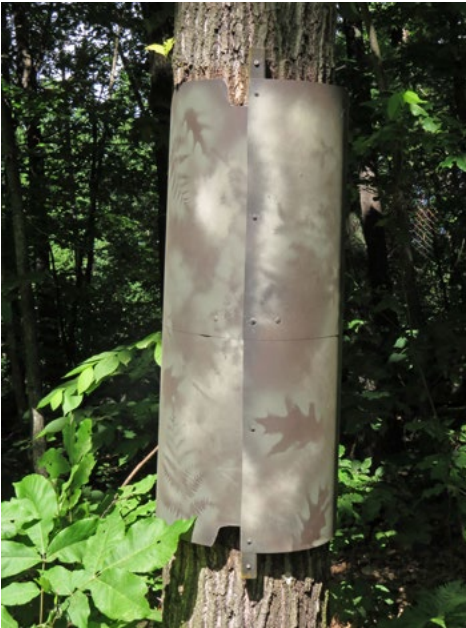
Close-up of flashing around tree trunk.
